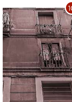
10 C. Pedreres Barcelona Sants-Montjuïc district
